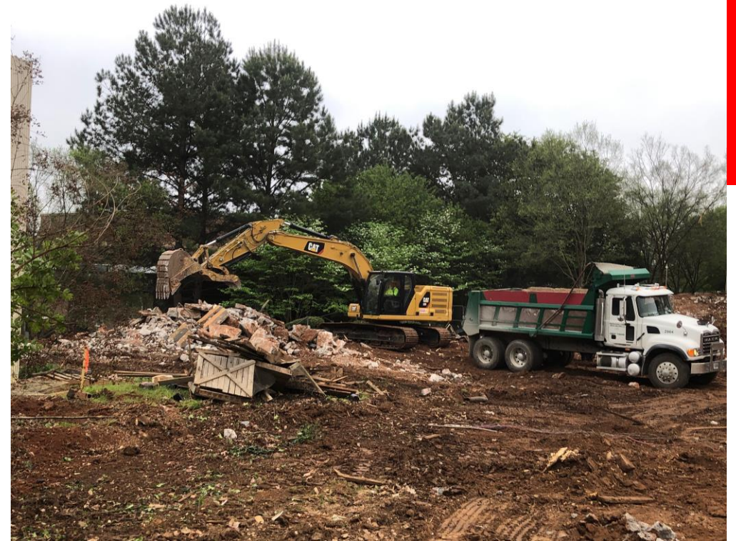
Removal of Debris and Unsuitable Soils
